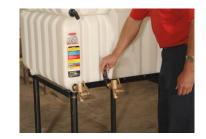
\*Again, sufficiently coat all threaded fittings with pipe thread sealant to prevent leakage.
