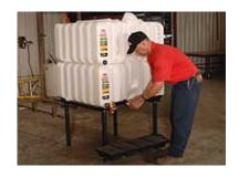
Install valve directly into bottom tank drain port. Install additional valves into elbow kits on stand.
