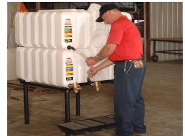
**Step 10:** Fill each tank. Be sure to double check each fitting for leaks. RTT is not responsible for fluid loss or clean up costs.
